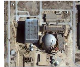
Picture 3: Ikonos Imagery of Iran Nuclear Reactor Construction, May 2001
