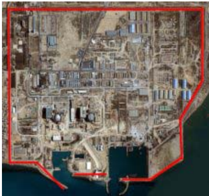
Picture 4: Ikonos Imagery of Iran Nuclear Reactor Construction, May 2001
